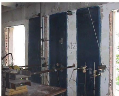
Figure 5: Representative Test Wall
