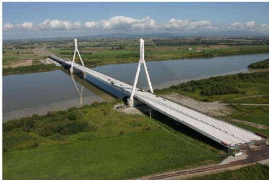
(a) Overview of bridge
