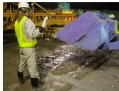
(c) Placement of HPFRCC
