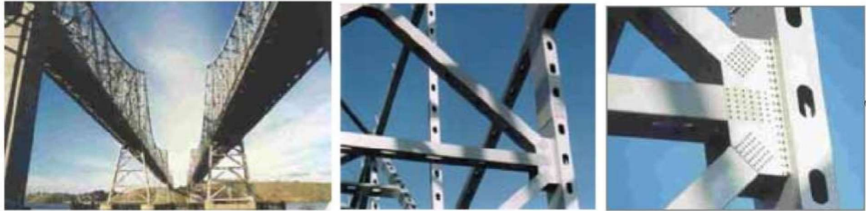
Figure 1.3. Double Gusset-Plate Connections of Carquinez Bridge Braced Frame Towers, Northern California
