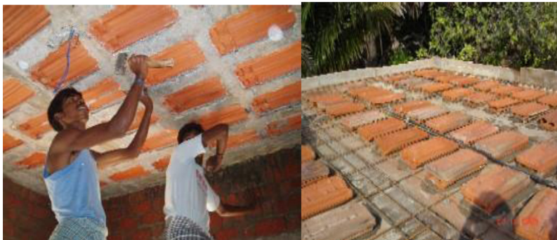
FIGURE 20.3 Reinforced cement concrete filler slab.
