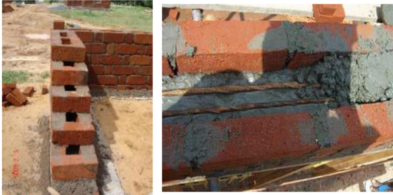
FIGURE 20.2 Rat-trap bond walling.
