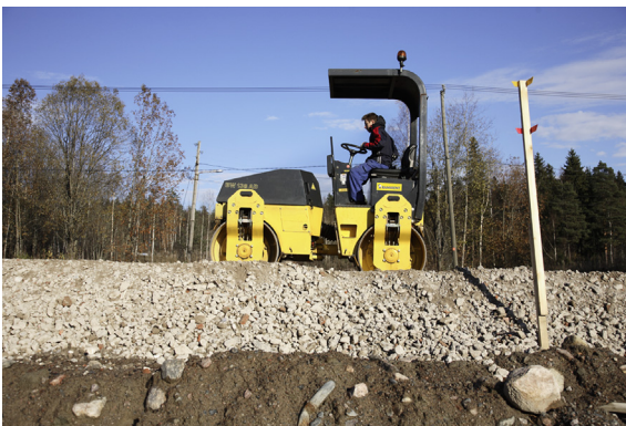
FIGURE 17.1 Road building using reclaimed concrete.
