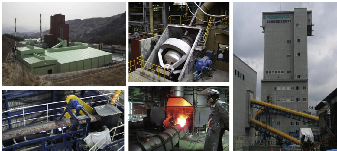
FIGURE 22.7 Top-submerged lance (TSL) and Kaldo technology for the recycling of copper and also e-waste and similar copper-containing materials ( www.outotec.com ).
