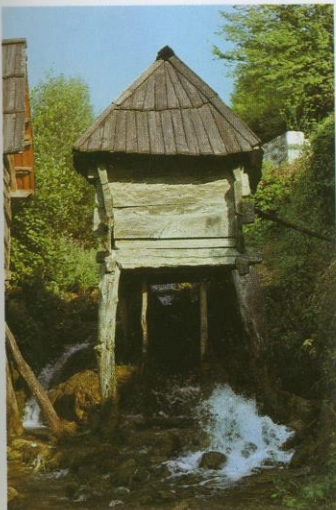
Water-mill ( below ) at Jajce, Bosnia. The water is channelled to gush against a horizontal paddle, which turns the millstone, here mounted in the wooden superstructure. (39)
