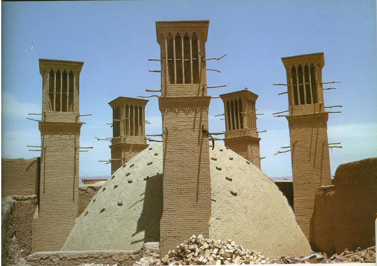
Ice-house ( below ) at Kerman, Iran. Ice, formed during frosty winter nights in shallow channels protected from the sun's rays by the high wall, is packed between layers of straw in the mud-brick dome. (40)
