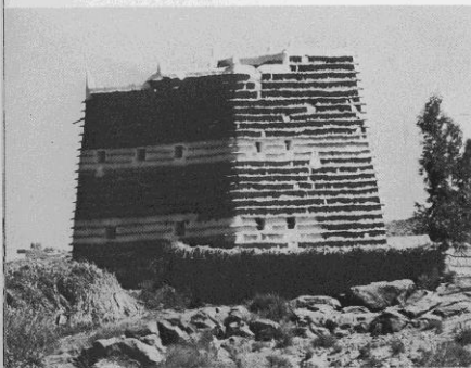
Saudi Arabia: in Abha, houses have successive mud courses separated by bands of downward projecting stones, to prevent the frequent rains from eroding the walls. (16)
