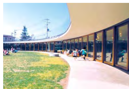
3. Children move around a semi-outdoor terrace that connects to the kindergarten building.
