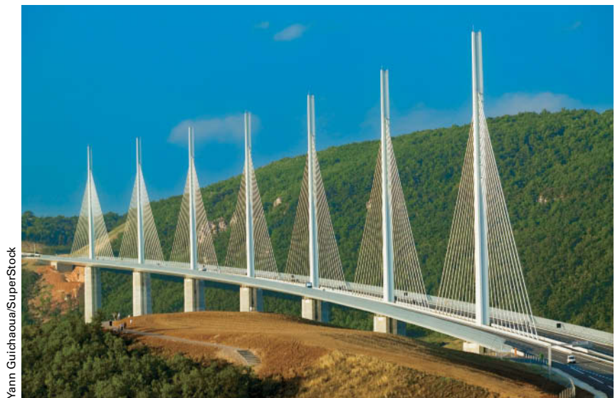
The Millau Viaduct in southern France. Note that the full height of the pylons is obscured here.
