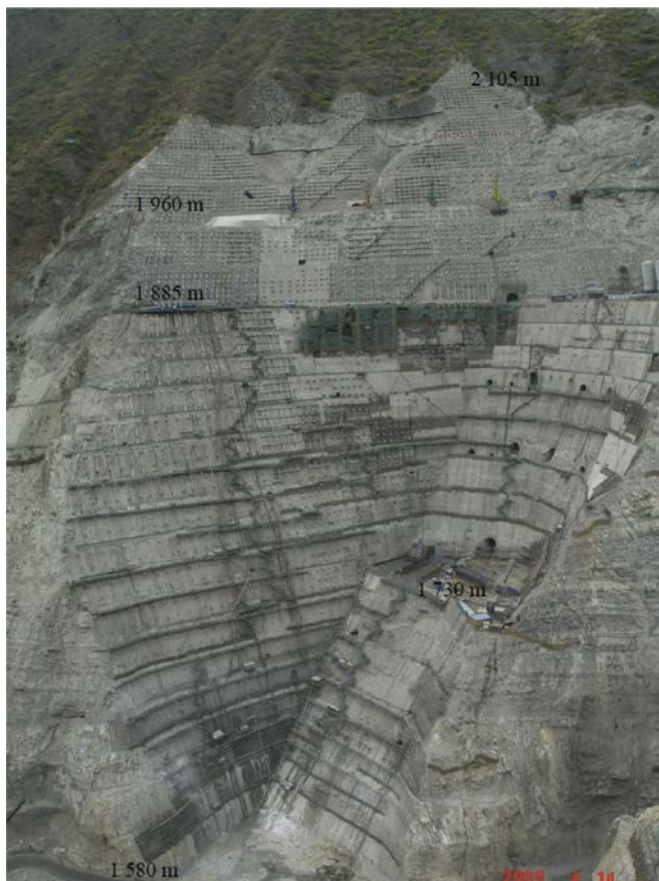
Fig. 8. The left abutment slopes of Jinping I hydropower station (Song et al., 2011).
