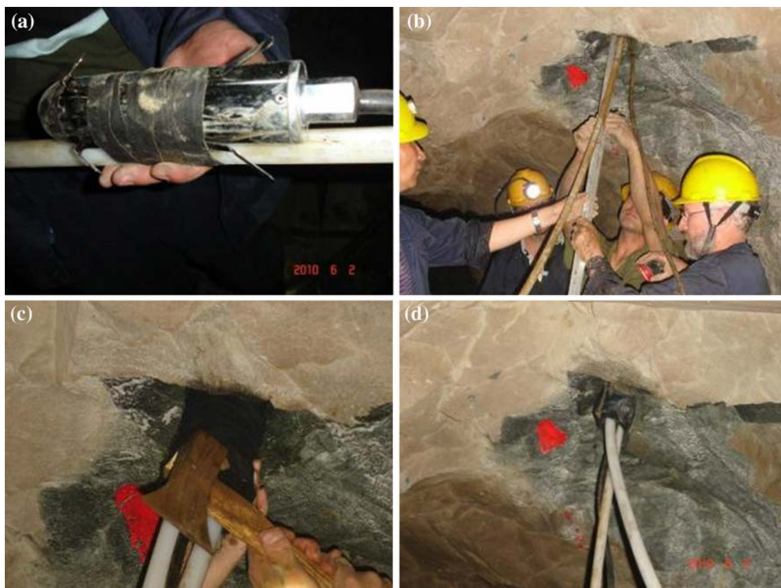
Fig. 11 The grouting installation process for a sensor in an upwardly inclined borehole: a tying the sensor and exhaust pipe together, b sensor is placed to the borehole bottom, c sealing of orifice, and d grouting
