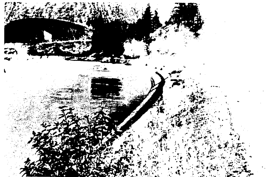
Figure 12.17. Seton Canal, secondary oscillations at wave front. (Courtesy of British Columbia Hydro and Power Authority, Vancouver, Canada).
