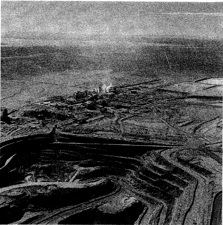
Figure 23.30: Mining and processing of borax at the US Borax Mine, Boron, California.
