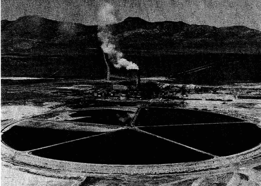
Figure 23.28: Crystallization of magnesium chloride on the shores of the Great Salt Lake, Utah (Amax).
