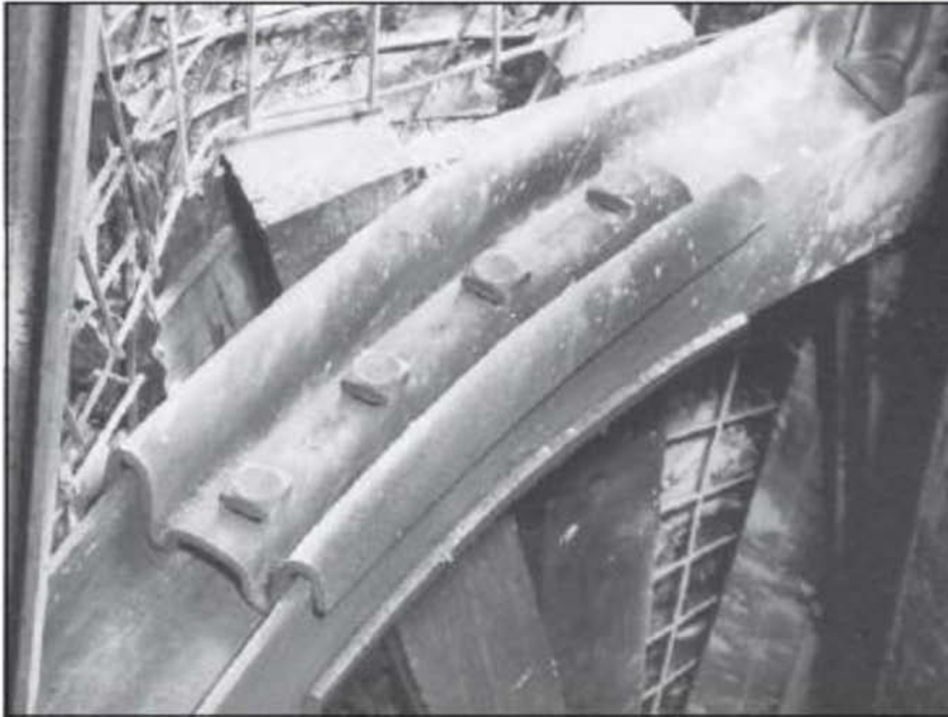
Figure 8-7-12 Wrap-around fishplate arch joint
