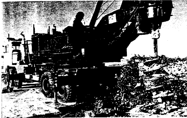
Figure 11.34 Spinning the auger to remove the cuttings (ADSC: The International Association of Foundation Drilling).
