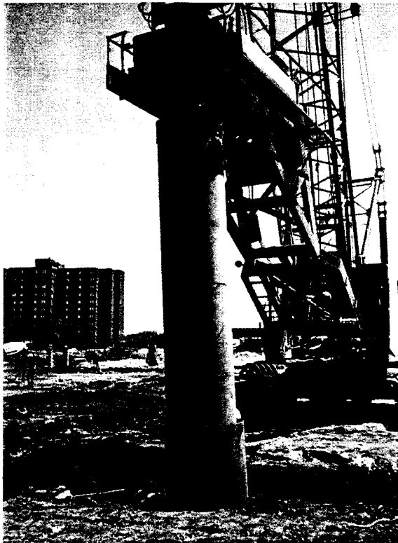
Figure 11.39 The contractor at this site is using casing. The first casing, visible at the bottom of the photograph, is already in place. However, its length is limited by the height of the rig. When casing must extend to greater depths, a second smaller casing is installed by passing it through the first casing, as shown here.
