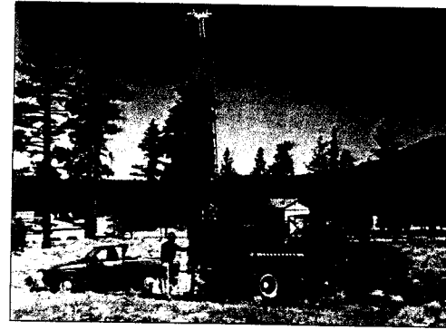
◀ Plate I Drilling an exploratory boring
