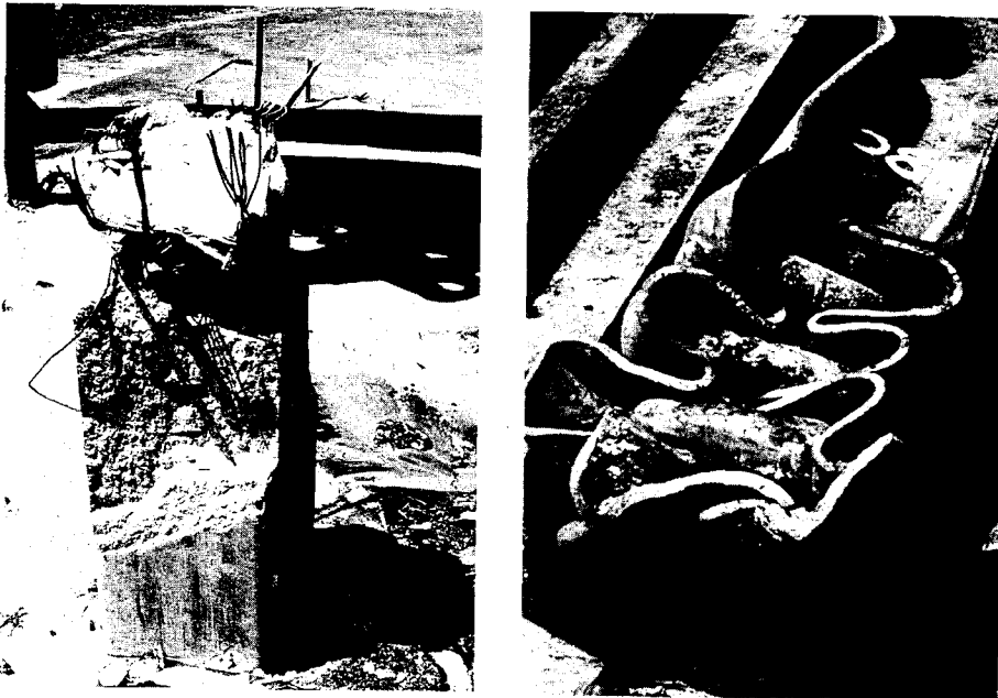
Figure 15.5 These piles were damaged during driving because the contractor selected a hammer that was too large. A driveability analysis could have predicted these problems, and would have helped the contractor select a more appropriate hammer. (Courtesy of Goble Rausche Likins and Associates, Inc.)
