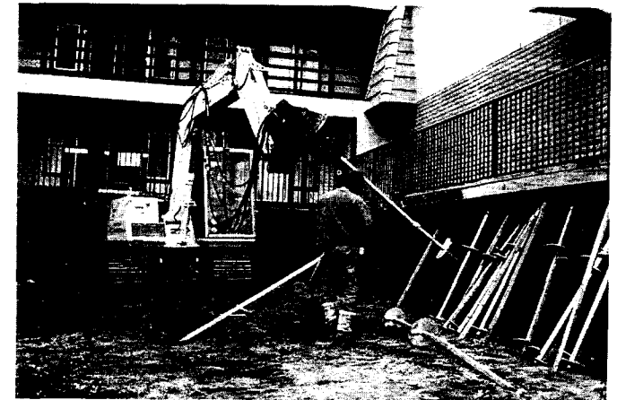
Figure 11.52 Installation of a helical anchor to be used as a tieback for a sheet pile wall. Once these anchors are installed, the soil in the foreground will be excavated (Photo courtesy of A. B. Chance Company).
