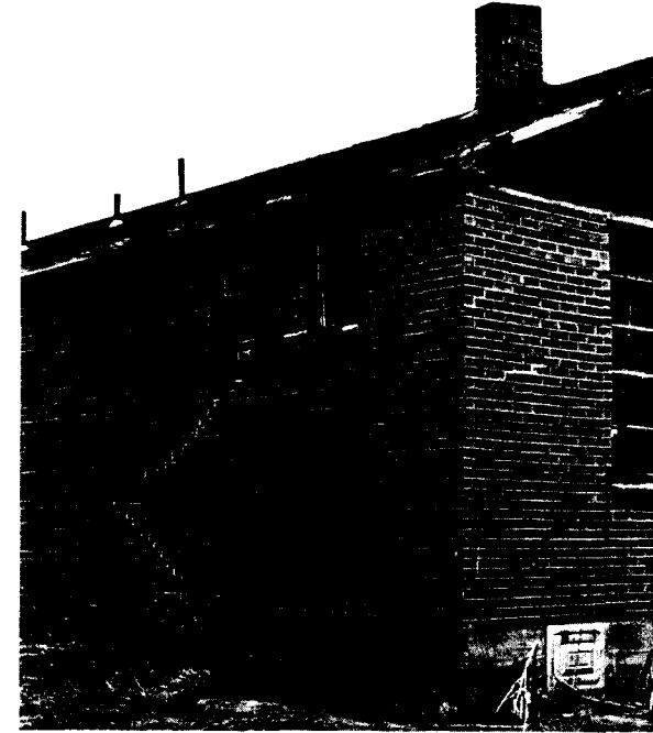
Figure 19.3 Expansive soil caused this brick building to crack (Photo courtesy of the Colorado Geological Survey).
