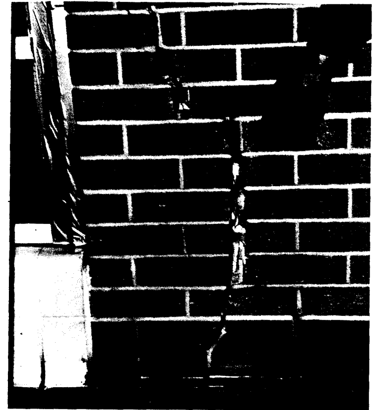
Figure 19.1 Heaving of an expansive soil caused this brick wall to crack. The $490,000 spent to repair this and other walls, ceilings, doors, and windows represented nearly one-third of the original cost of the six-year-old building (Photo courtesy of the Colorado Geological Survey).
