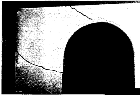
◀ Plate E Cracks in the interior walls of a house that experienced excessive differential settlements
