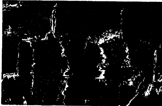
Figure 24.23 Moisture migration through this retaining wall has caused unsightly water stains. a) overall view of wall; b) close-up view. This problem could have been avoided by use of proper waterproofing or dampproofing behind the wall.
