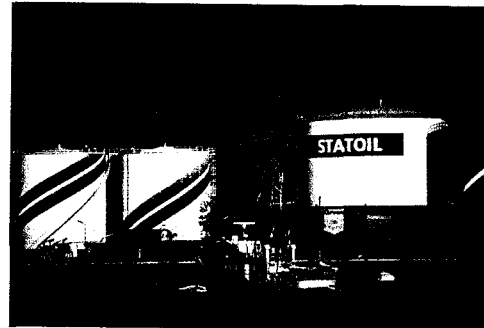
▲ Plate C Petroleum storage tanks
