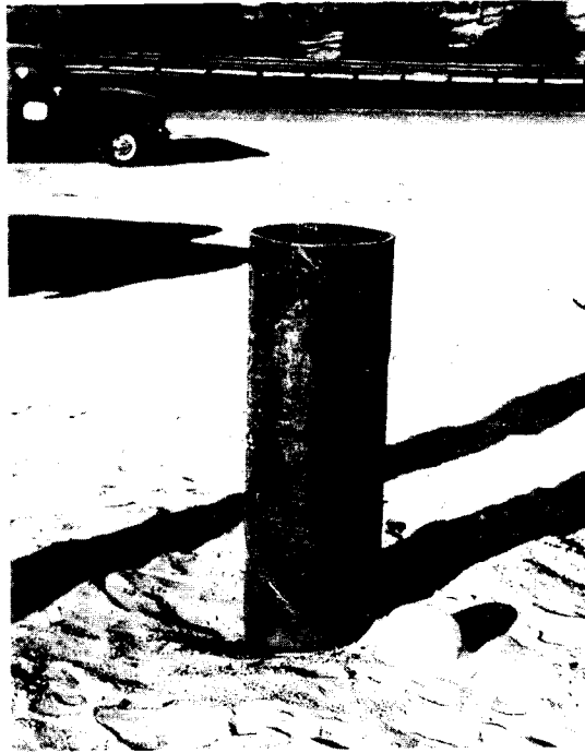
Figure 11.10 A 16 inch (406 mm) diameter steel pipe pile.
