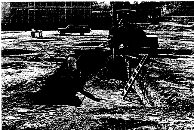
Figure 5.6 A backhoe making an excavation for a spread footing.
