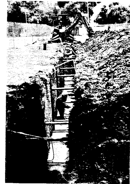
Figure 4.7 This exploratory trench was dug by the backhoe in the background, and has been stabilized using aluminum-hydraulic shoring. An engineering geologist is logging the soil conditions in one wall of the trench.
