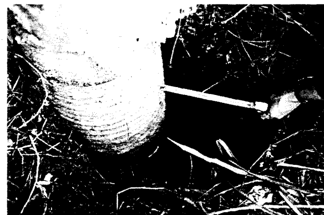
Figure 17.5 This pile, which supported a bridge near Watsonville, California, moved laterally during the 1989 Loma Prieta Earthquake, creating a gap between the pile and the soil. The size of this gap is an indication of the excessive lateral deflections that occurred during the earthquake (Loma Prieta Collection, Earthquake Engineering Research Center, University of California, Berkeley).
