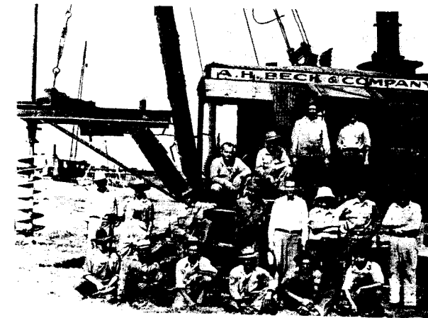
Figure 11.29 Early truck mounted drill rig and crew, circa 1925 (ADSC: The International Association of Foundation Drilling).
