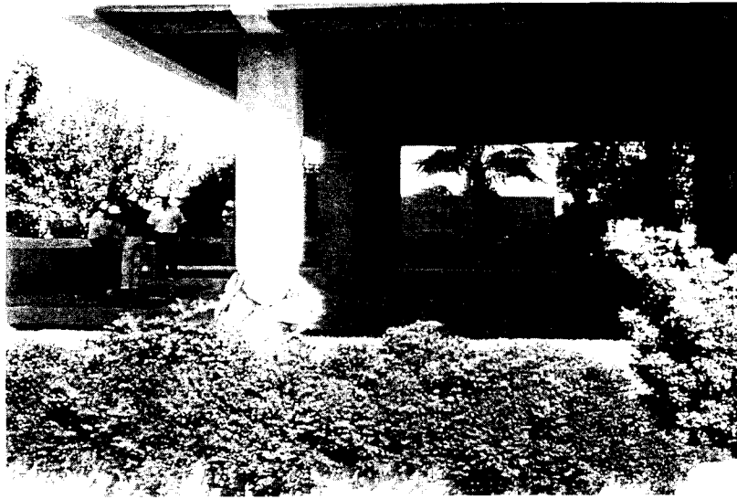
Figure 9.21 Imperial County Services Building, El Centro, California. The bases of these columns failed during the 1979 El Centro earthquake, causing the building to sag about 300 mm. As a result, this six-story building had to be demolished. (U.S. Geological Survey photo)
