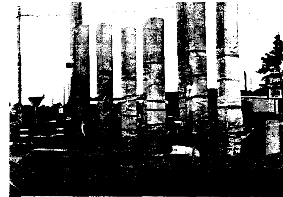
Figure 18.3 These prestressed concrete piles will support a bridge abutment. They extend above the ground surface because the abutment fill has not yet been placed. Since the underlying soils are compressible, and will settle due to the weight of the fill, the piles have been wrapped with lubricated polyethylene sheets to reduce the downdrag forces between the piles and the fill. The next stage of construction will consist of building a mechanically stabilized earth (MSE) wall around these piles and backfilling it to approximately the height of the piles (Photo by Dr. Kamal Tawfiq).
