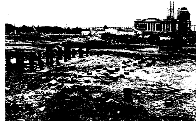
Figure 11.4 Groups of timber piles. Those in the foreground have been cut to the final head elevation (National Timber Piling Council).
