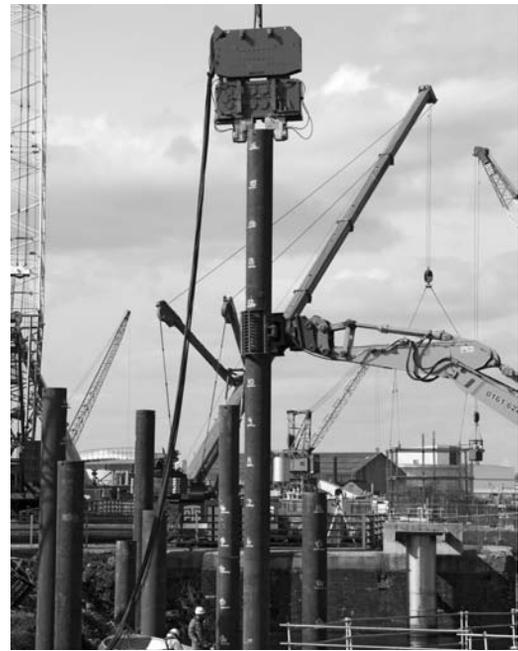
**Figure 9.7** (continued) Pile-driving equipment: (e) vibratory pile driver; (f) photograph of a vibratory pile driver (Courtesy of Reinforced Earth Company, Reston, Virginia)
