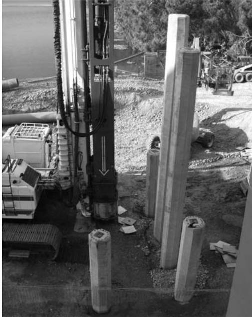
**Figure 9.45** Driving of piles in a group
