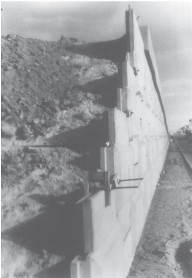
**Figure 13.24** Reinforced-earth retaining wall (with metallic strip) under construction
