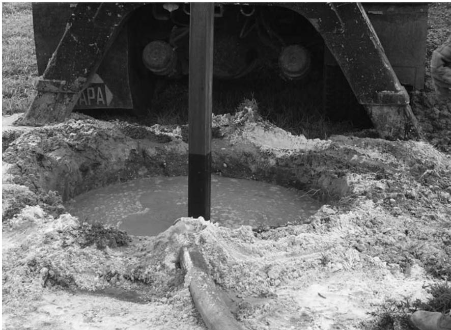
**Figure 10.6** Drilled shaft construction using wet method (Courtesy of Khaled Sobhan, Florida Atlantic University, Boca Raton, Florida)
