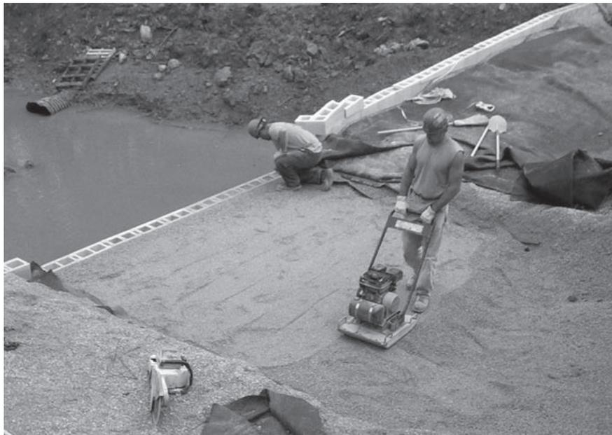
**Figure 13.32** Construction of a geotextile-reinforced retaining wall (Courtesy of Jonathan T. H. Wu, University of Colorado at Denver, Denver, Colorado)
