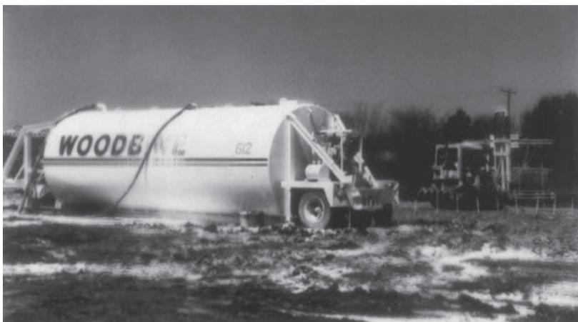
**Figure 11.23** Pressure injection of lime slurry for a building pad (Courtesy of Hayward Baker Inc., Odenton, Maryland.)
