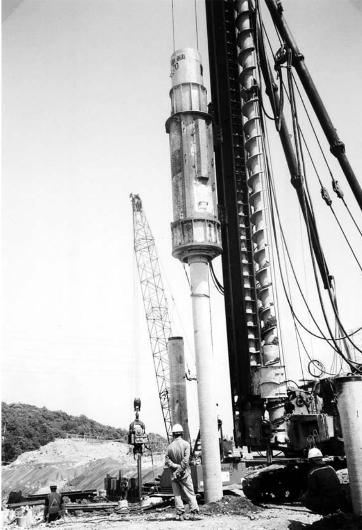
**Figure 9.8** A pile-driving operation in the field (Courtesy of E. C. Shin, University of Incheon, Korea)
