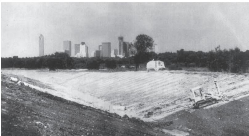
**Figure 11.24** Slope stabilization of a canal bank by pressure injection of lime–fly-ash slurry (Courtesy of Hayward Baker Inc., Odenton, Maryland.)
