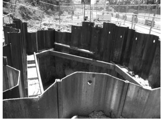
**Figure 14.5** A small enclosure with steel sheet piles for an excavation work (Courtesy of N. Sivakugan, James Cook University, Australia)
