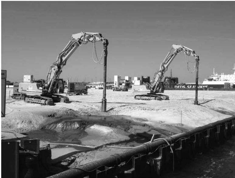
**Figure 16.32** Construction of a stone column [DGI-Menard (USA).]
