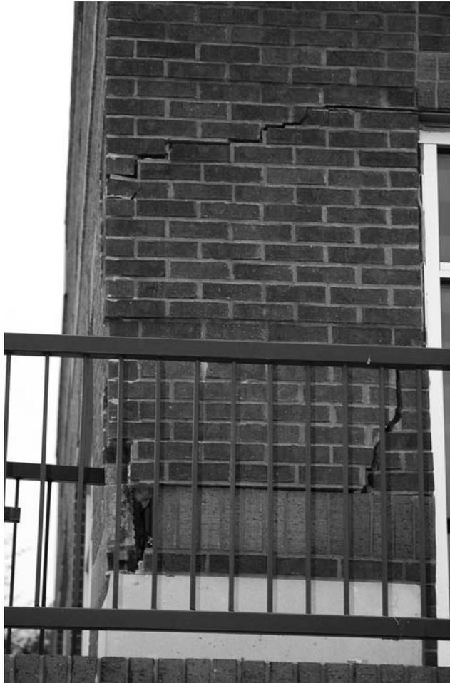
**Figure 11.8** Cracks in a wall due to heaving of an expansive clay (Courtesy of Anand Puppala, University of Texas at Arlington, Arlington, Texas)
