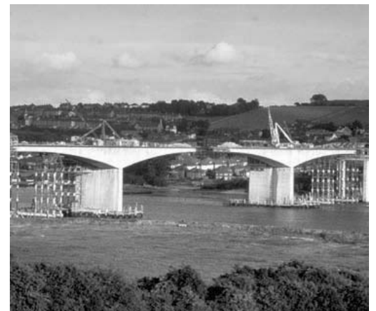
Photo 5.2 Nonprismatic cantilever beams of bridge during construction.
