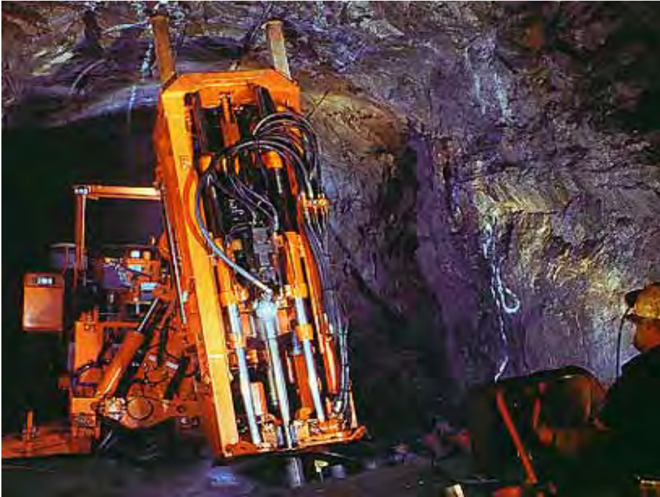
Remotely operated rig drilling into a stope
