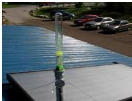
The bubble separator of a bubble-pump system
