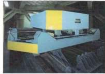
Tuned mass damper for Chiba-Port Tower.
