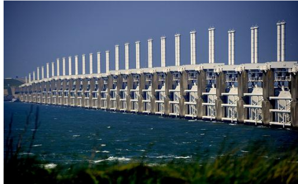
شکل (۸-۱) storm surge barrier in Eastern Scheldt
